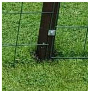
If the fence is going to be erected in a straight line and the end panel is too long simply bend the panel at right-angles to the exact length, do NOT cut the panel down.
