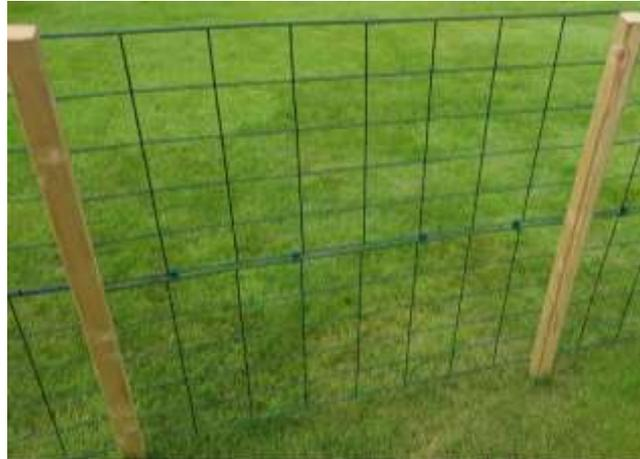
Check the fence for alignment and level. You can now trim the fence posts level with the top of the panels if you require but this is up to your own preferences.
